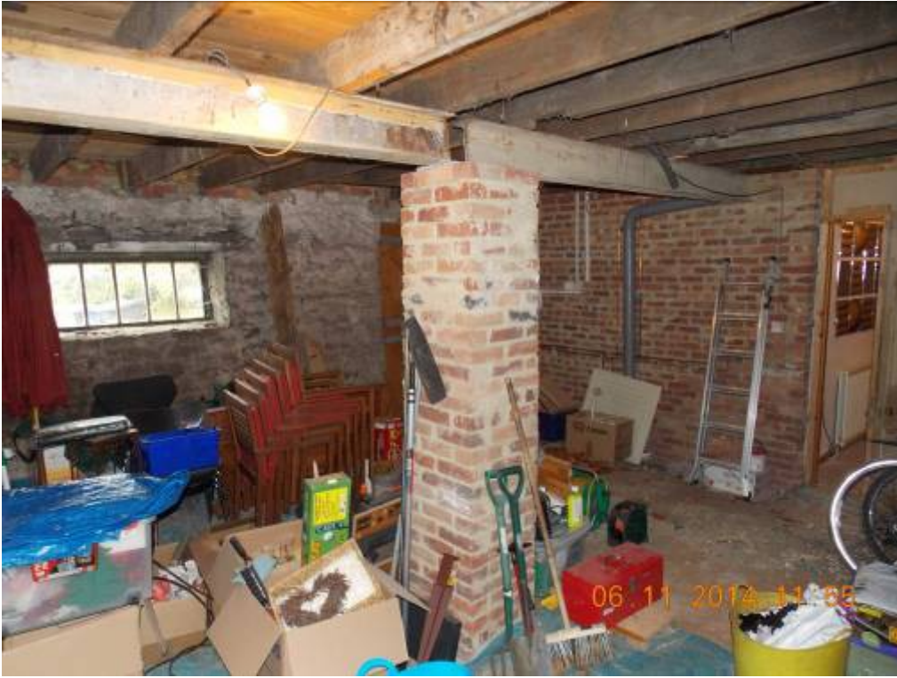
Existing masonry pier and steel beam
