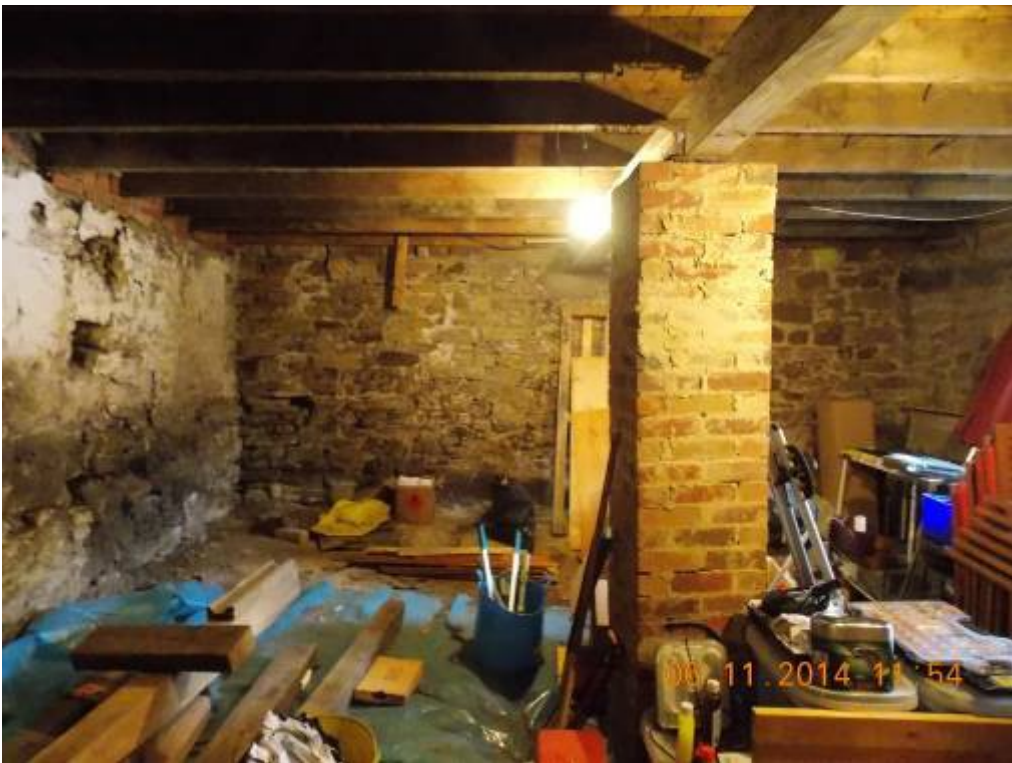
Existing masonry pier and steel beam
