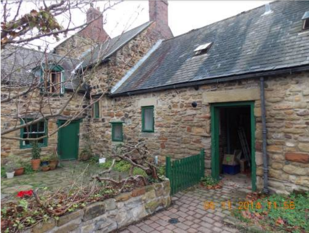
Rear elevation and back door to undeveloped space
