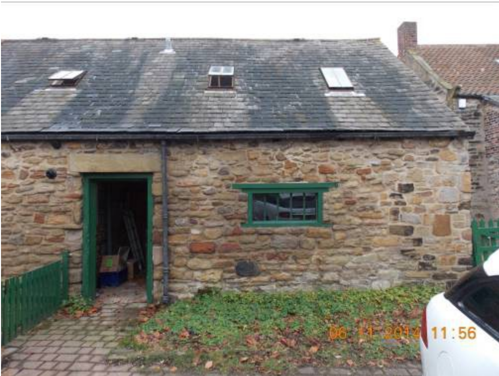
Rear elevation and existing window into undeveloped space
